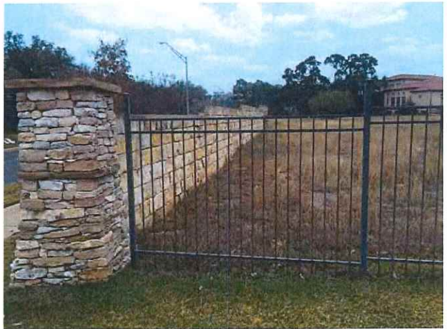
Fence Type "A" and "B" Corner
